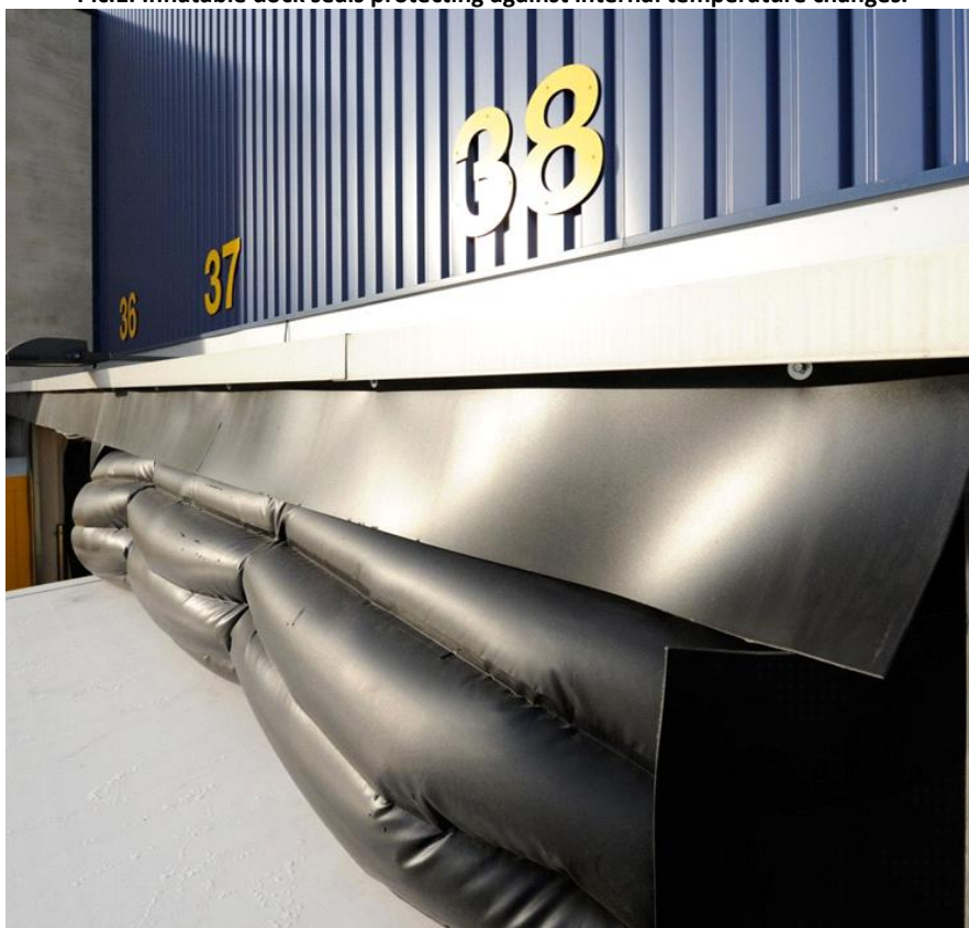
Pic.1. Inflatable dock seals protecting against internal temperature changes.
